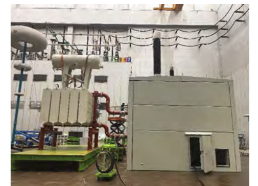
Figure 4 | Test of the structure of the soundproof room
