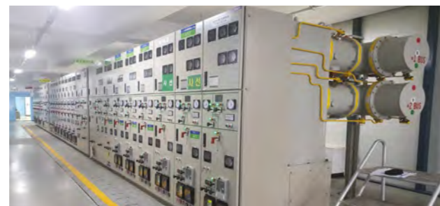
Figure 1 | Installed DAIS Product
